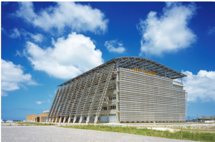
City hall equipped with a solar energy generation system on the roof and the wall facing south (Itoman City, Okinawa Prefecture)
